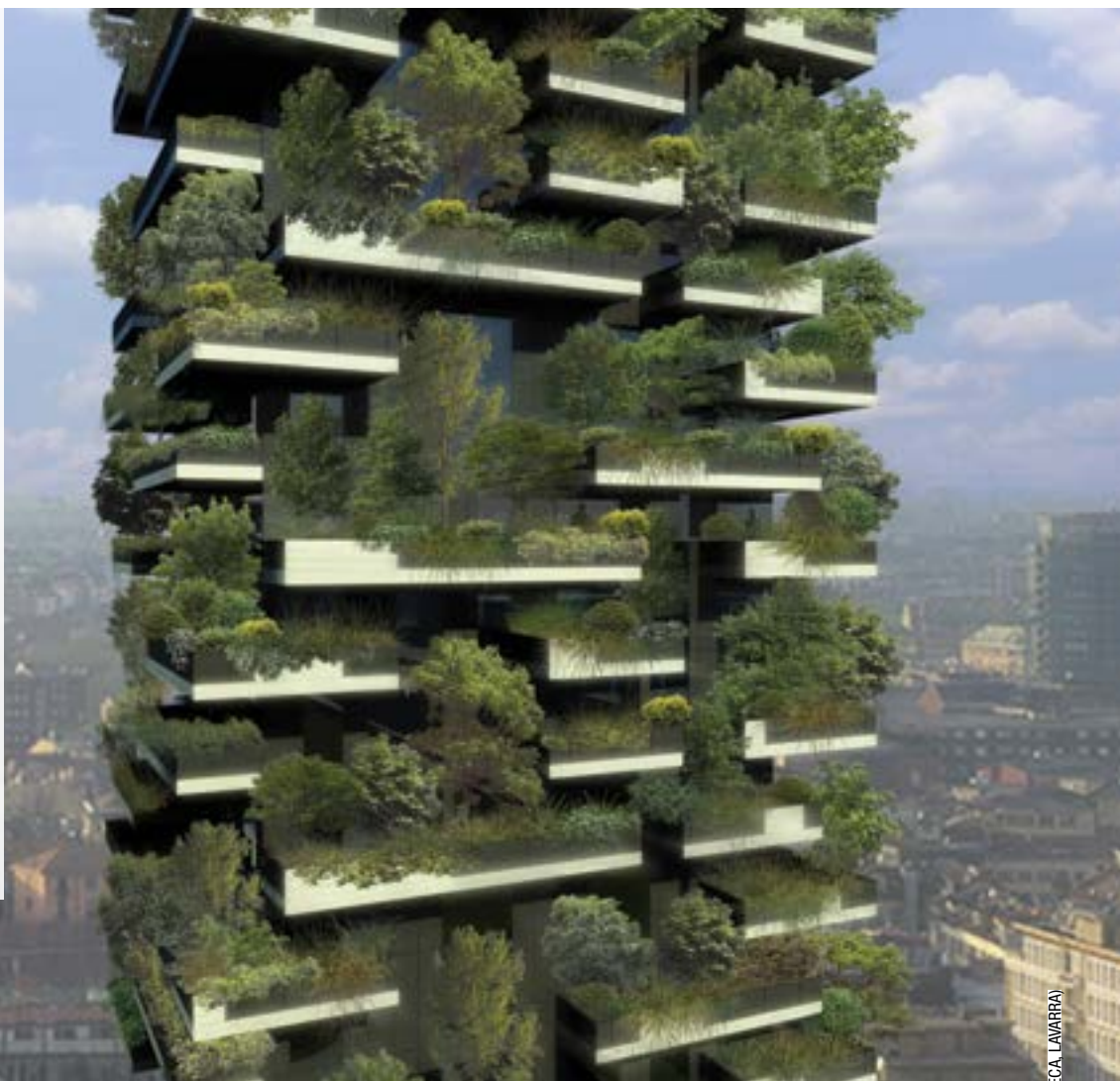
LIMB LIFE Think of the apartment complex as the planet's first intuitively smart urban tree house, deliberately planted with species that moderate temperatures with the season and with a self-sustaining gray water irrigation system.
